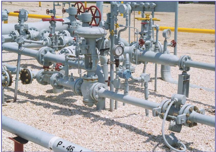
A common meter-run setup.
