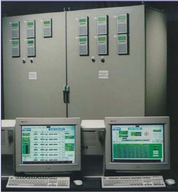
**Installation of flow computers communicating to a PLC system within a control room environment.**
