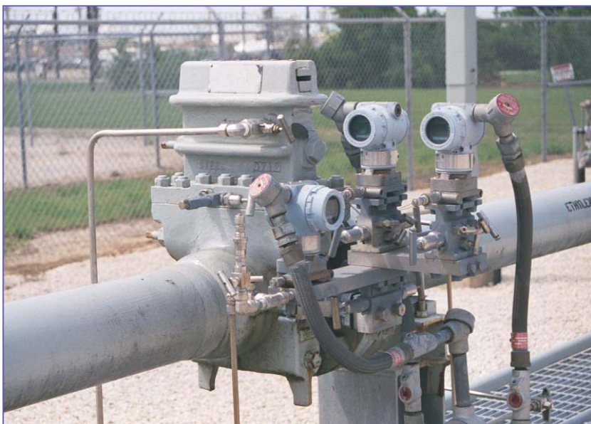
Using a field mounted transmitter as a secondary transducer to the primary flow meter.
